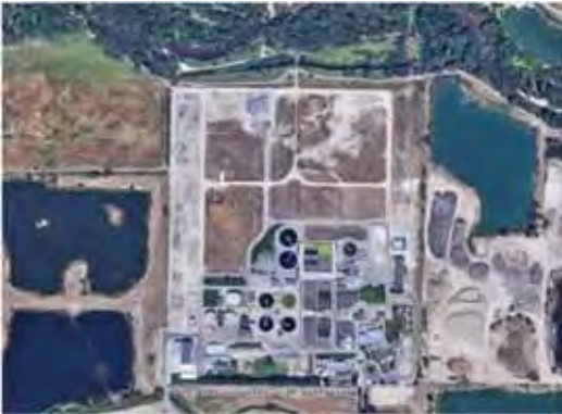
West Boise Water Renewal Facility
